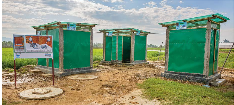
▲ Humanitarian aid also includes building toilet blocks, as here in Bangladesh.
