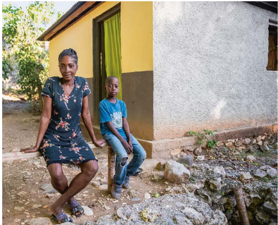
▲ Jesula Pierre (49) and her son Franklin (9) live in a stone house built by Diakonie Katastrophenhilfe following the 2010 earthquake in Binet, Sud-Est department, Haiti.
